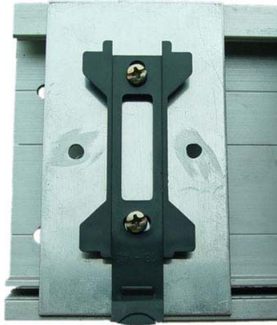
Fix the bracket and Aluminum board on the S7-300 PLC rail
